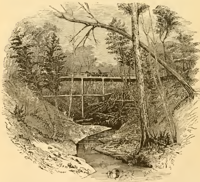
HIGH BRIDGE, LAKE BLUFF, LAKE COUNTY, ILLINOIS.
